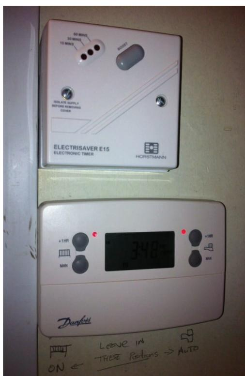
**Figure 1(a).** Hot water boost (top) and main control with handwritten instruction to leave in set positions (below)
