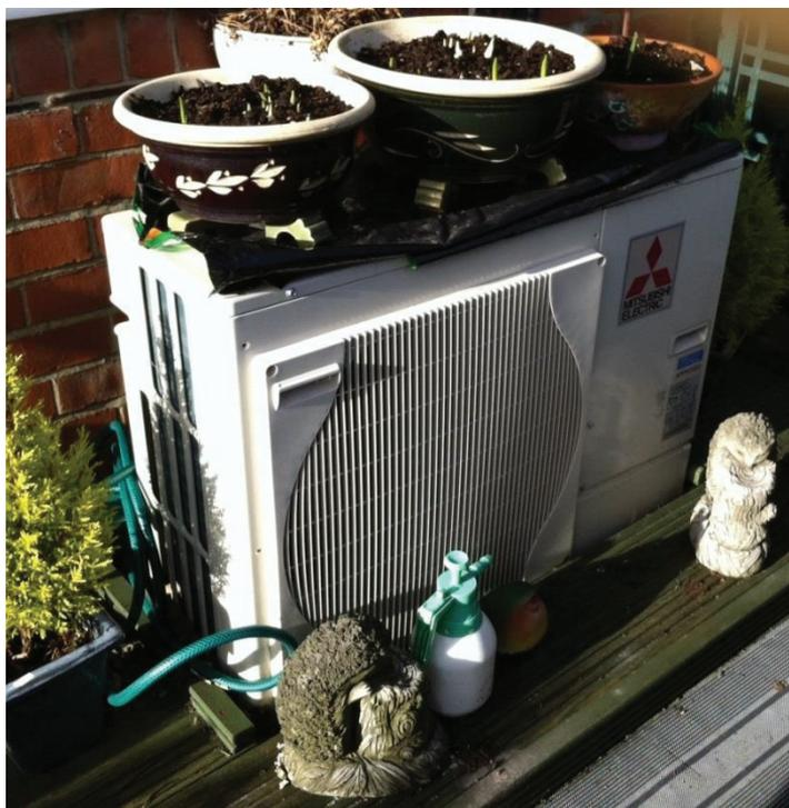
**Figure 2.** Air source to water heat pump external unit, South Tyneside, showing new elements being fitted into the existing physical external space. This example indicates how integration between the old and the new extends beyond the immediate energy related practices such as heating, washing and ventilation, to other activities such as gardening.
